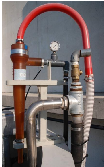
FIGURE 2: HYDROCYCLONE ON THE DEMON ® PILOT TO RETAIN ANAMMOX AND REMOVE COMPETING BACTERIA SUCH AS NITRITE-OXIDIZING BACTERIA AND ANOXIC HETEROTROPHIC BIOMASS
