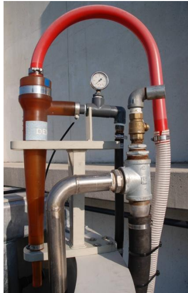
FIGURE AI-2: HYDROCYCLONE TO RETAIN ANAMMOX AND WASH OUT COMPETING BACTERIA
