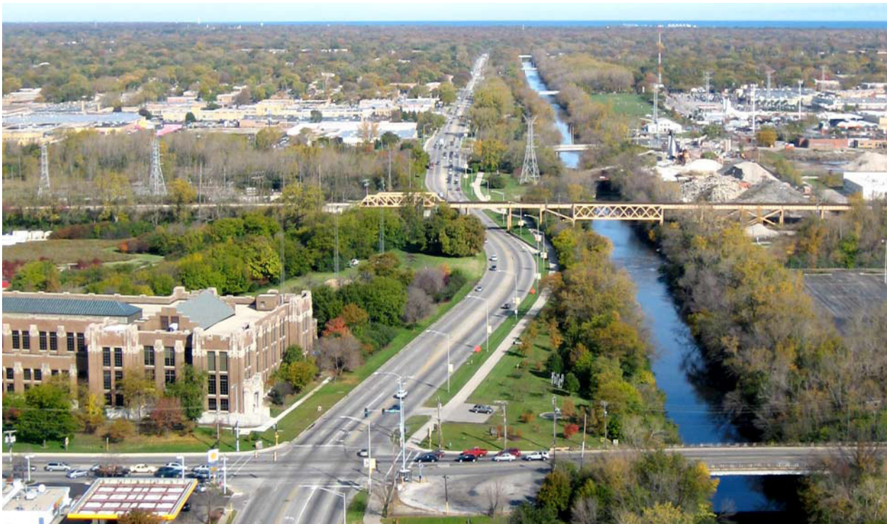
Photograph 1 : Aerial view of the North Shore Channel with Howard Street Bridge in the foreground.
