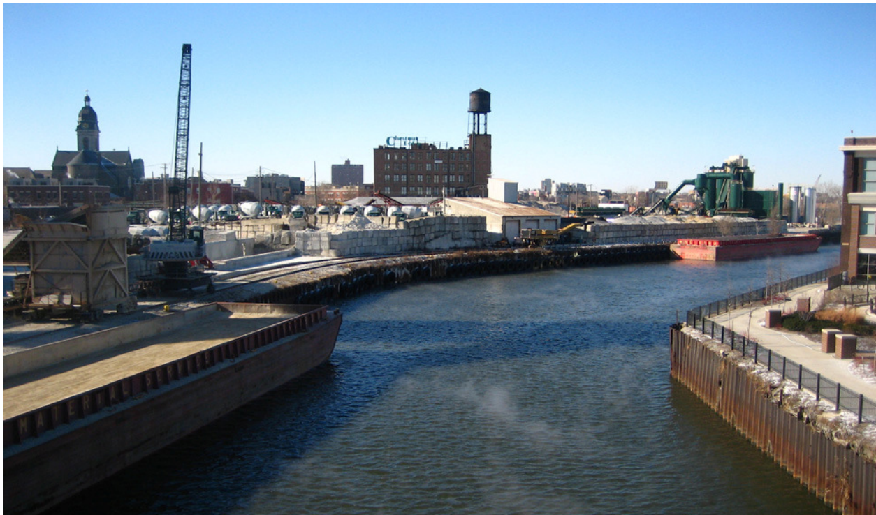
Photograph 2: North Branch Chicago River, west from Halsted Street Bridge.
