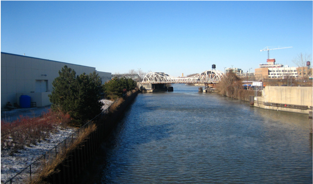
Photograph 3: North Branch Canal, northwest from Halsted Street Bridge.
