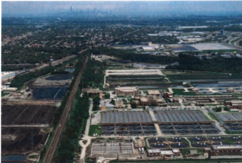
The Calumet plant, where MWRD will expand its anaerobic digester to save energy. The digesters are in the foreground. (Metropolitan Water Reclamation District)
