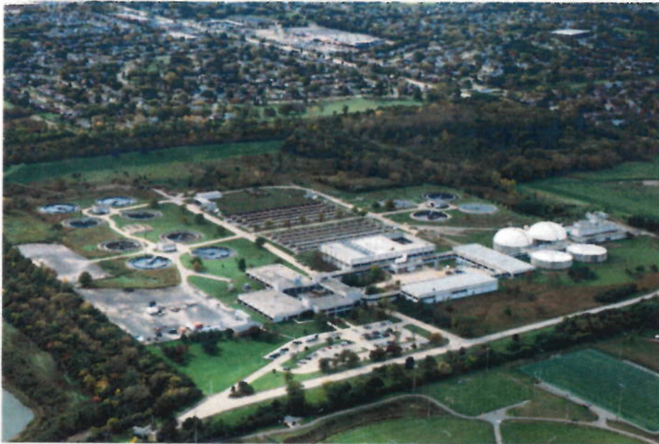
Before and after aerial images of the Metropolitan Water Reclamation District of Greater Chicago's Egan Water Reclamation Plant looking southwest show how the plant has been a staple while the surrounding Schaumburg community sprawled with development between 1975 and 2015. Communities come to rely on water treatment facilities like Egan, and the closer the plant, the quicker the water is cleaned.
