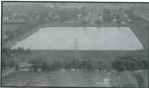
Structure 86. Northlake Reservoir.
