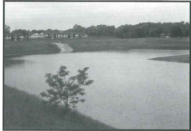
Widespread residential flood damages (left) can be reduced or eliminated by structural measures such as floodwater storage reservoirs (right).
