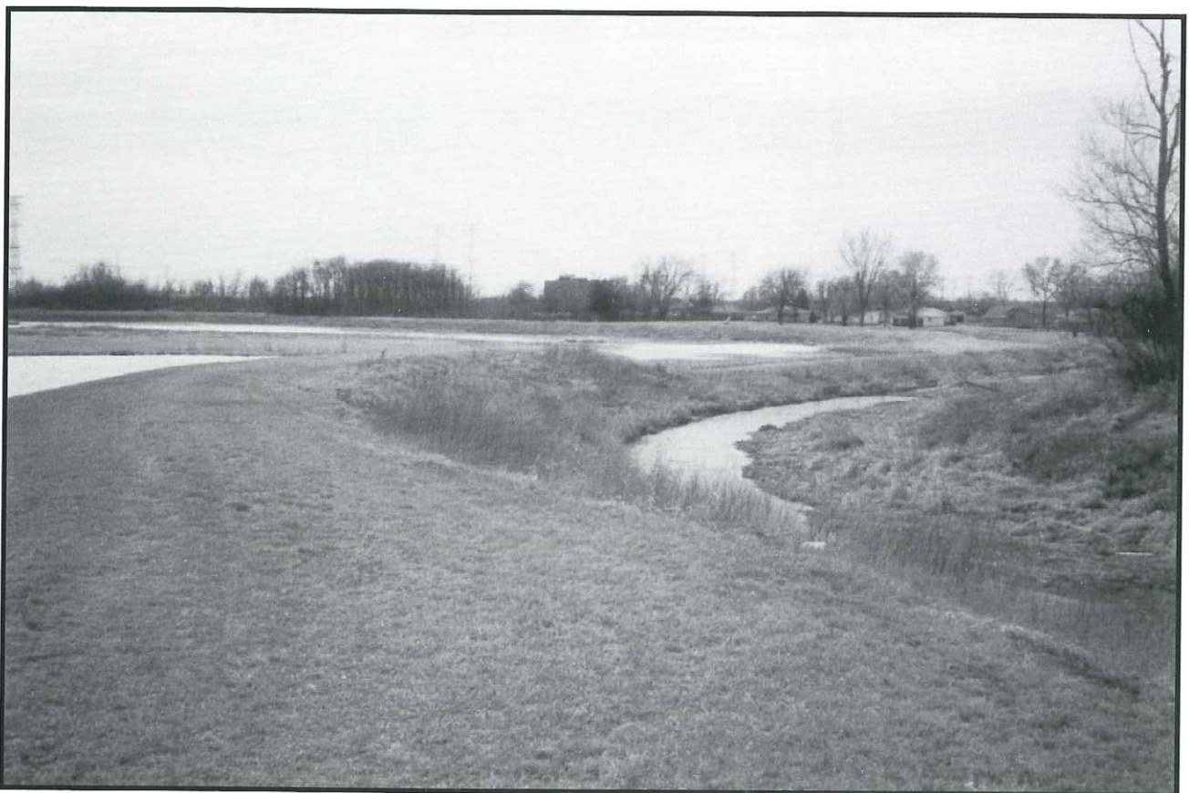
Salt Creek Channel Improvement.
