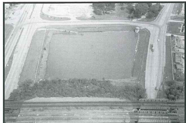
Eugene A. Doyle Reservoir; Lake Street Reservoir
