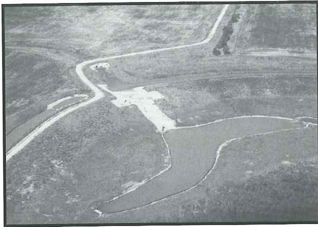
Northbrook Reservoir, Structure 32-A. July 1981
