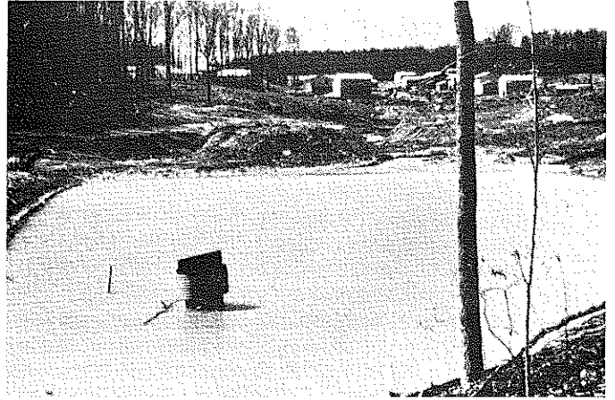
Besides the loss of valuable top-soil, lack of proper erosion protection measures during and after any construction work will produce sediment (left), a major factor in increased flood levels. Techniques like the sediment trap shown (right) will reduce or eliminate this unnecessary condition.
