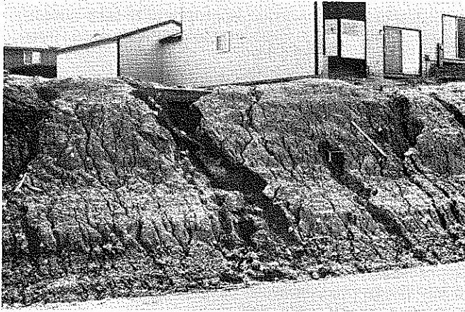
Besides the loss of valuable top-soil, lack of proper erosion protection measures during and after any construction work will produce sediment (left), a major factor in increased flood levels. Techniques like the sediment trap shown (right) will reduce or eliminate this unnecessary condition.
