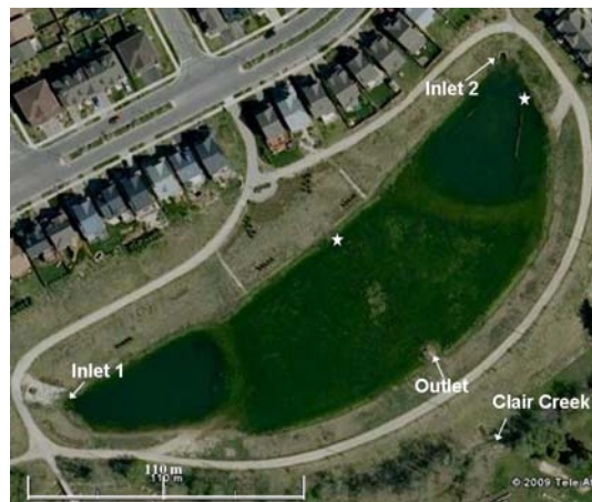
Figure 17. Aerial photograph of Pond 45.
