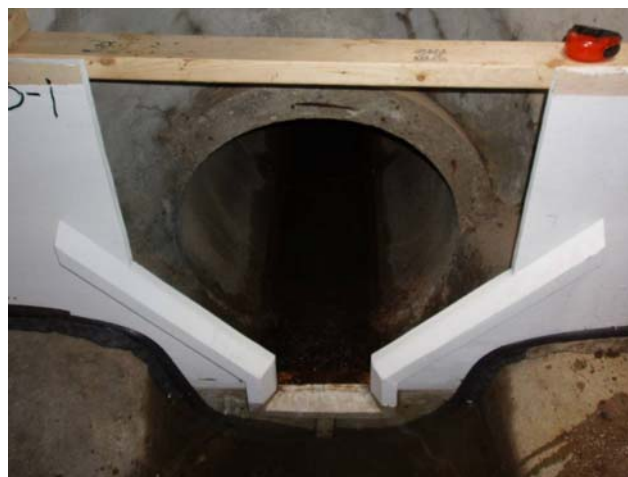
Figure 38. Compound Weir Installed
