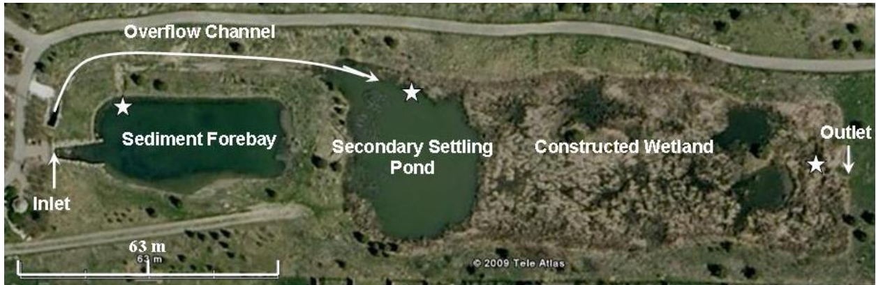
Figure 16. Aerial photograph of Pond 33.
