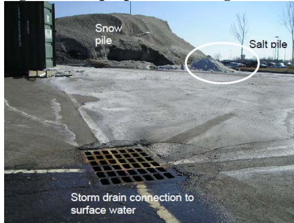
Figure 26. Improper Site Management
