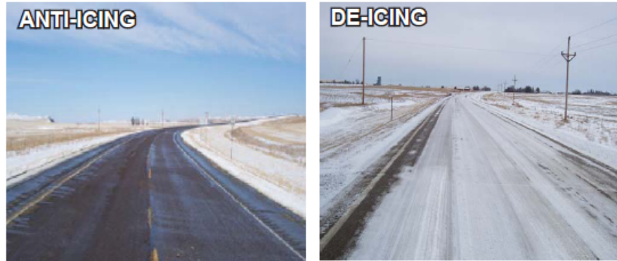
Figure 31. Road Conditions Anti-Icing vs. De-Icing
