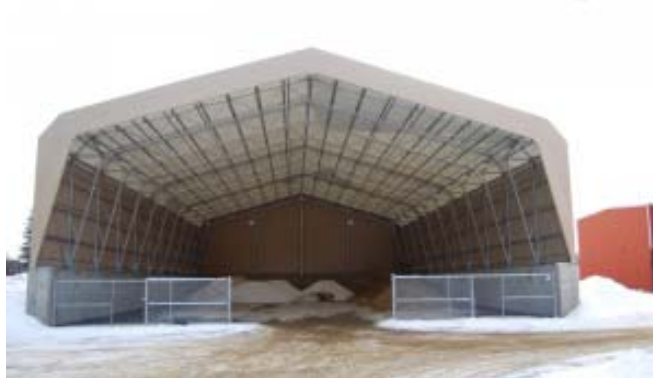
Figure 27. Town of Derry NH Salt Storage
