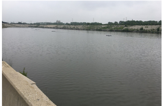
The McCook Reservoir Stage I filled in June, demonstrating a fully operational system retaining water that formerly discharged to the Chicago Area Waterways System or ended up in basements of homeowners and businesses. Another 6.5 billion gallons of capacity will become available through Stage II.
