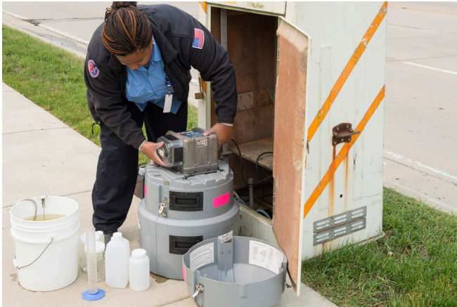
Pollution Control Technician Candace Bays services an automatic sampler and collects wastewater samples from an industrial user located in the Kirie WRP's drainage basin.
