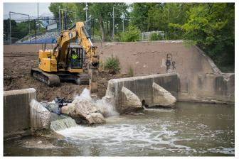
An earthmover begins removing the MWRD's 108 year old dam to improve the flow of the North Shore Channel.
