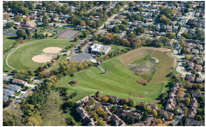
The Mayfair Reservoir Expansion Project in Westchester provides direct flood reduction benefits to about 60 residential structures and reduces storm-related impacts for approximately 120 homeowners.
