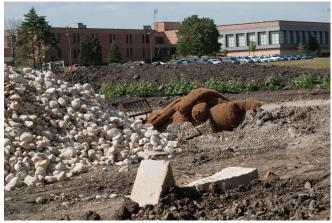
Gravel riffle stones pile up in front of Homewood-Flossmoor High School as a part of the Cherry Creek East Branch flood control project that includes the construction of an overflow channel. The stones provide instream habitat for aquatic organisms.
