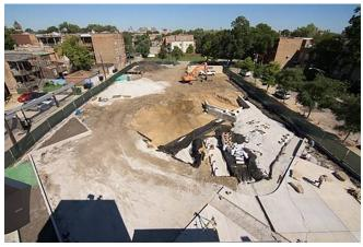
Crews have demolished more than 34,000 square feet of impervious asphalt pavement, 1,000 square feet of concrete pavement and 2,400 square feet of playground rubber tiles at Wadsworth Elementary School as part of the Space to Grow program.
