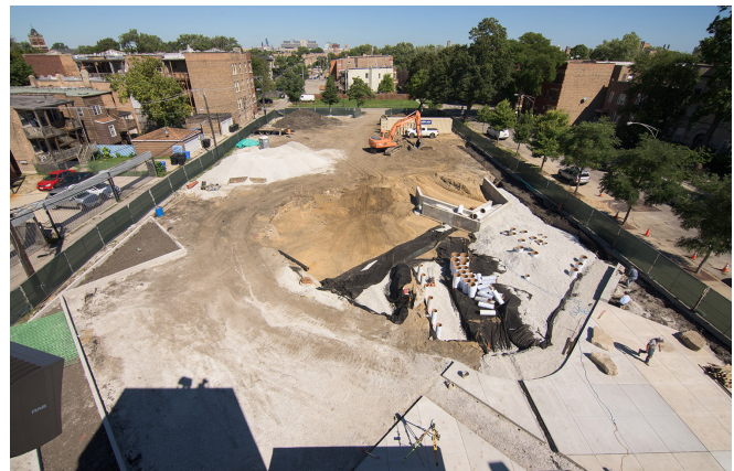
Wadsworth Elementary School construction.
