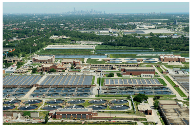
The sprawling Metropolitan Water Reclamation District of Greater Chicago’s Calumet Water Reclamation Plant, 400 E. 130th St., treats on average 354 million gallons of water per day to serve Chicago and 48 south suburbs.
