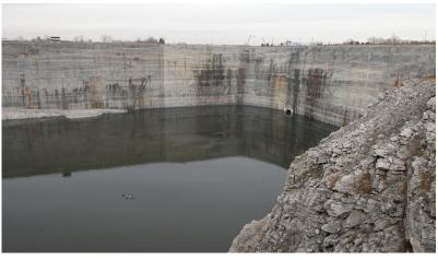
Completed in 2015, Thornton Composite Reservoir has a storage capacity of 7.9 BG and is the largest combined sewer reservoir in the world. The reservoir, with a surface area of approximately 83 acres, serves a 90-square-mile area in Cook County. The reservoir provides an estimated \$40 million per year in flood control benefits to 556,000 people in 14 communities, including the South Side of Chicago and 13 suburban communities.
