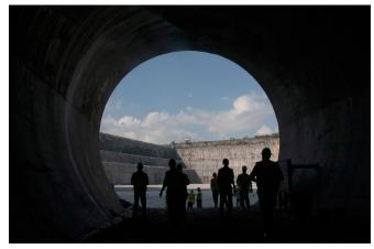
The final connection between the tunnel and Thornton Reservoir receives heavy traffic once steady rain hits the Chicago area. Water will stream out of the tunnel at velocities of up to 30 feet per second before being pushed back into the tunnel on an incline to be treated at the Calumet Water Reclamation Plant.
