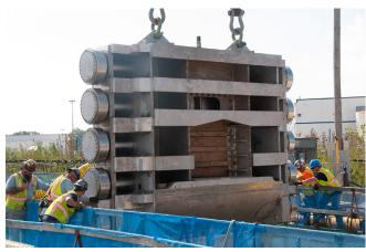
Earlier this year, crews placed a 100-ton stainless steel gate into the bottom of the tunnel connection to the Thornton Composite Reservoir, approximately 300 feet below ground. Workers had to meticulously install the gates by crane to fit precisely into the tunnels leading 1,300 feet to the reservoir.
