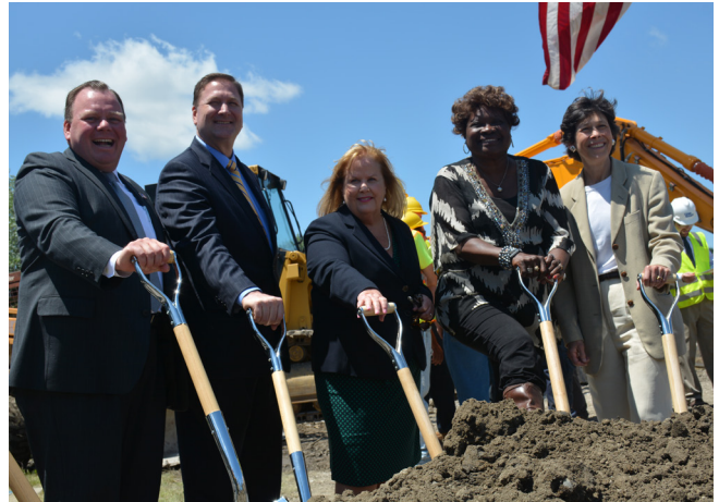
MWRD Commissioner Patrick D. Thompson, Exec. Director David St. Pierre, Pres. Kathleen Meany, Vice Pres. Barbara McGowan and Commissioner Debra Shore help break ground on an Oak Lawn project that will receive $12.7 million in low-interest loan assistance immediately as part of their nine-project Regional Water System Improvement program.
