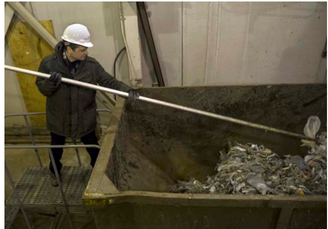
Congressman Quigley "raking down the dumpster" in the West Side Coarse Screen Building. The screens in this facility remove large objects, sticks, rocks, and tree branches that can cause damage to the pumps at the facility. This task needs to be done every few hours on a normal flow day, hourly during storms.
