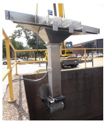
The MWRD worked with the Illinois Sustainable Technology Center to install an experimental prototype waterfall turbine in one of the Stickney Water Reclamation Plant's effluent channels. The turbine produces 1,200 watts of electricity from the falling water, which offers a small but important step towards energy neutrality.
