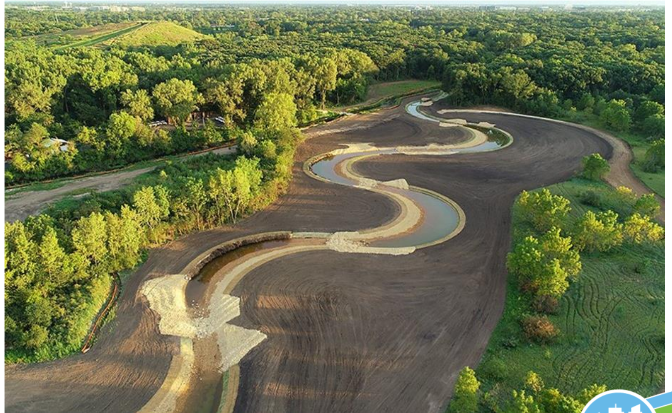
Photo: Forest Preserve District of DuPage County
