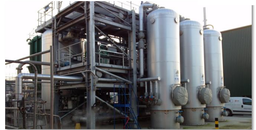
Thermal Hydrolysis System at Crawley WWTP (Image courtesy Cambi)
