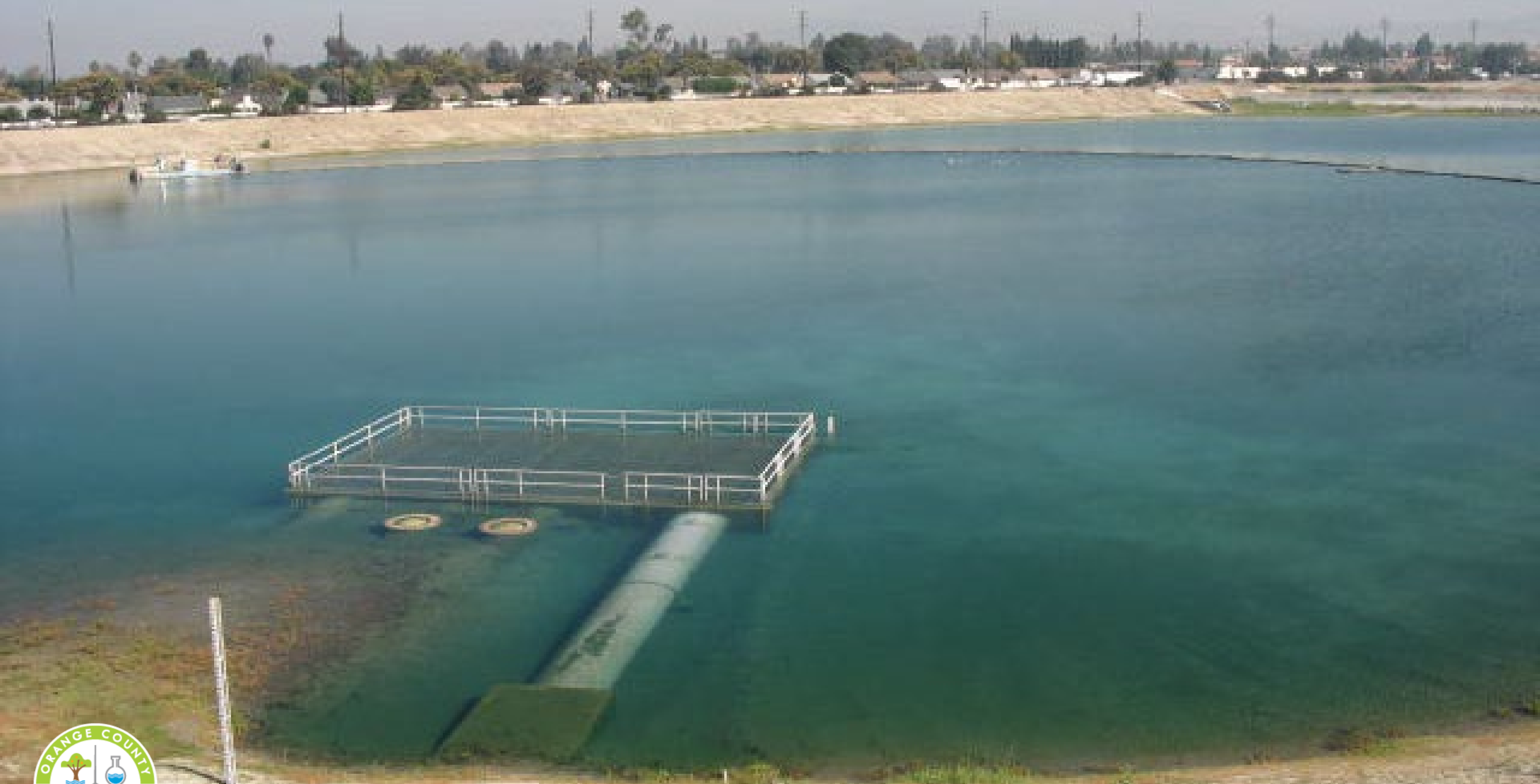
Basin with Submersible Pump Station
