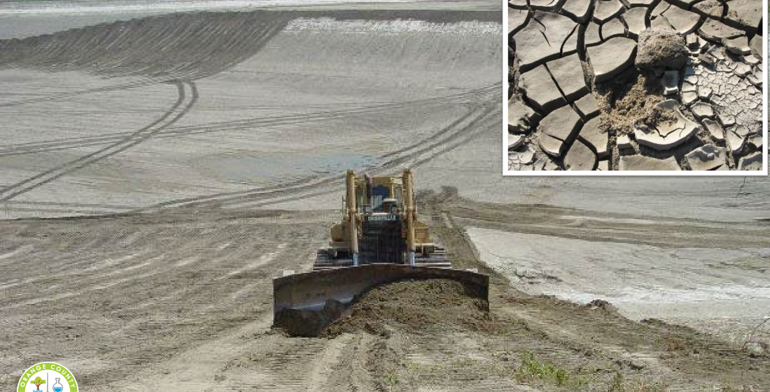
Heavy Equipment Cleans Recharge Basins
