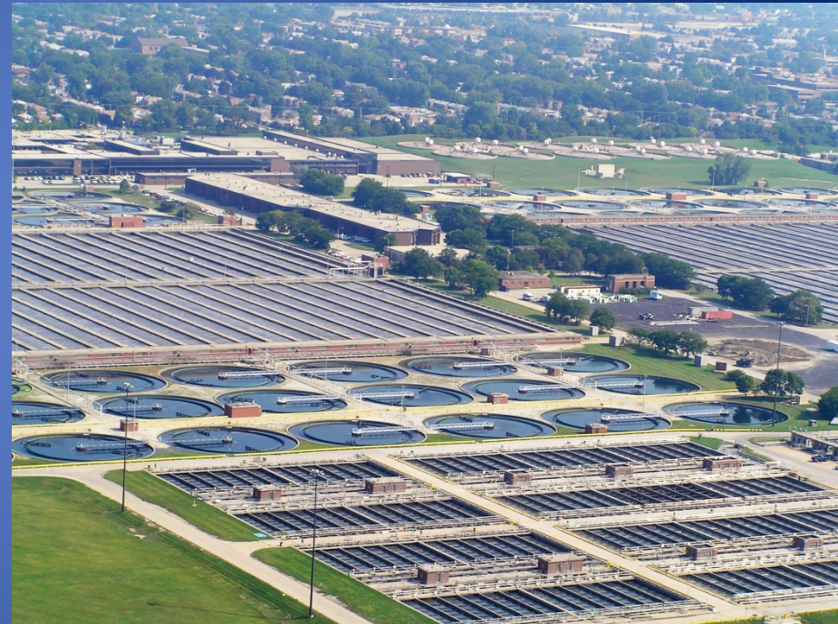
Stickney WWTP – 1.2 billion gal/day
