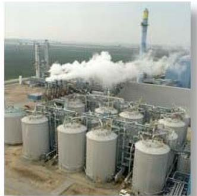
Photo courtesy of Industrial Innovations
