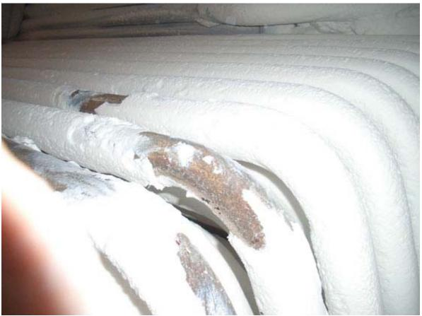
The sand-like material is SiO2 produced through oxidation (burning) of the volatized siloxanes contained in the digester gas. Figure shows siloxane deposition on boiler tubes.
