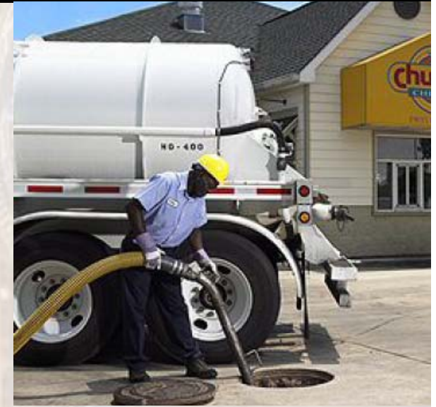
Grease Interceptor (Outdoor, In-ground)
