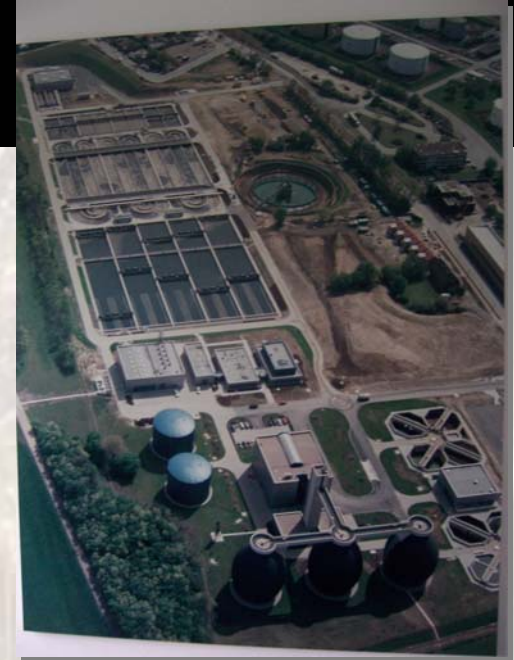
DU-Kasslerfeld WWTP, FOG Receiving & Storage
