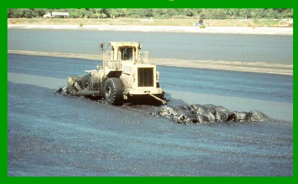
Rail System Pulled by a Bulldozer On Paved Drying Cells
