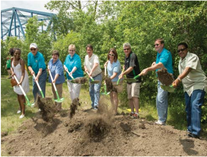
Local and state officials scoop up dirt to signify the beginning of construction on a portion of the Cal-Sag Trail in Alsip in June. Government officials, bicyclists, hikers and neighbors gathered in Alsip's Freedom Park for the groundbreaking. Fifty percent of the land has been set aside by the MWRD, and once complete, the trail will be 26 miles long.
