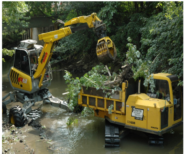
MWRD crews worked for more than 3 weeks during the summer of 2009 removing debris and vegetation along the North Branch of the Chicago River. The efforts were aimed to help prevent flooding and to stabilize the banks of the river.
