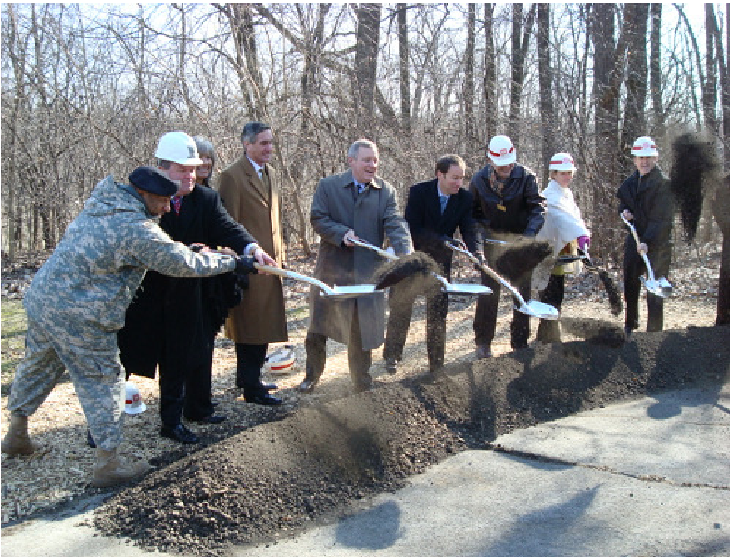
MWRD President Terrence J. O'Brien (second from left) and other officials commence kick off of the Levee 37 Ground breaking ceremony in March 2009 in Cook County Forest Reserve #2. The levee will provide flood protection for numerous businesses and more than 600 residential buildings, and is the result of 20 years of collaboration between the MWRD and the Army Corps, Illinois Department of Transportation, the villages of Mount Prospect and Prospect Heights, the Illinois Department of Natural Resources and the Forest Preserve of Cook County.
