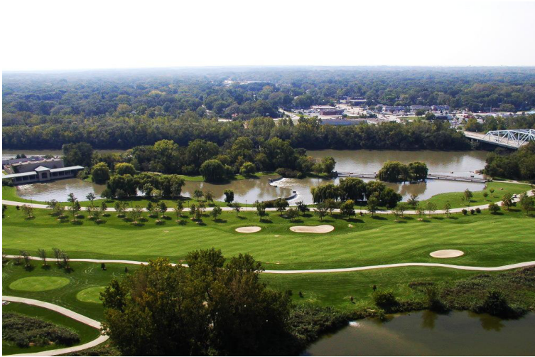
The District produces nearly 267,100 dry tons of biosolids each year, making its operation the largest in the country. The District has improved its final processing of biosolids to achieve over a 90% beneficial utilization of the product. Here, built next to a Sidestream Elevated Pool Aeration station, is Water's Edge Golf Course, developed with District biosolids.
