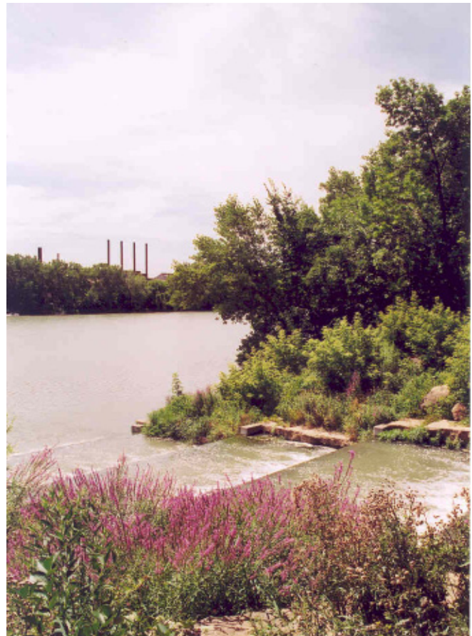
This Sidestream Elevated Pool Aeration Station (SEPA) has improved the quality of the water in the Calumet-River by introducing oxygen during the warm months of each year.
