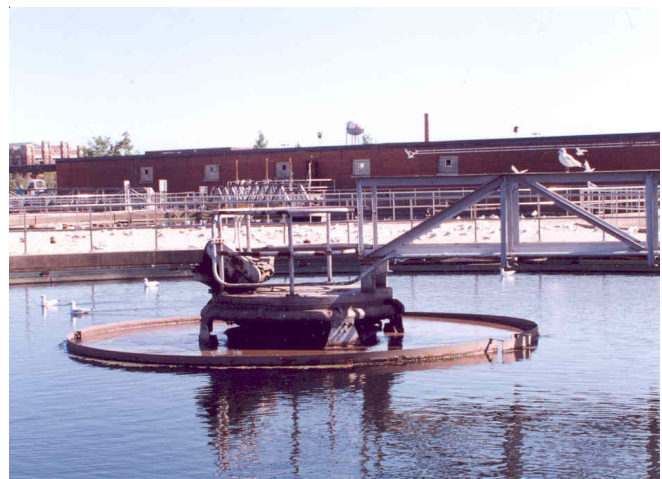
The Metropolitan Water Reclamation District operates seven wastewater plants in Cook County. More than one billion gallons of wastewater flow into the plants on an average day, and the treatment process removes 95% of the organic pollutants. This photo shows a final settling tank after the wastewater has undergone primary and secondary treatment. The effluent is released back into a receiving stream at the end of the process. The biosolids that were removed are disposed of in an environmentally safe manner. All seven plants consistently meet the limits of their operating permits.
