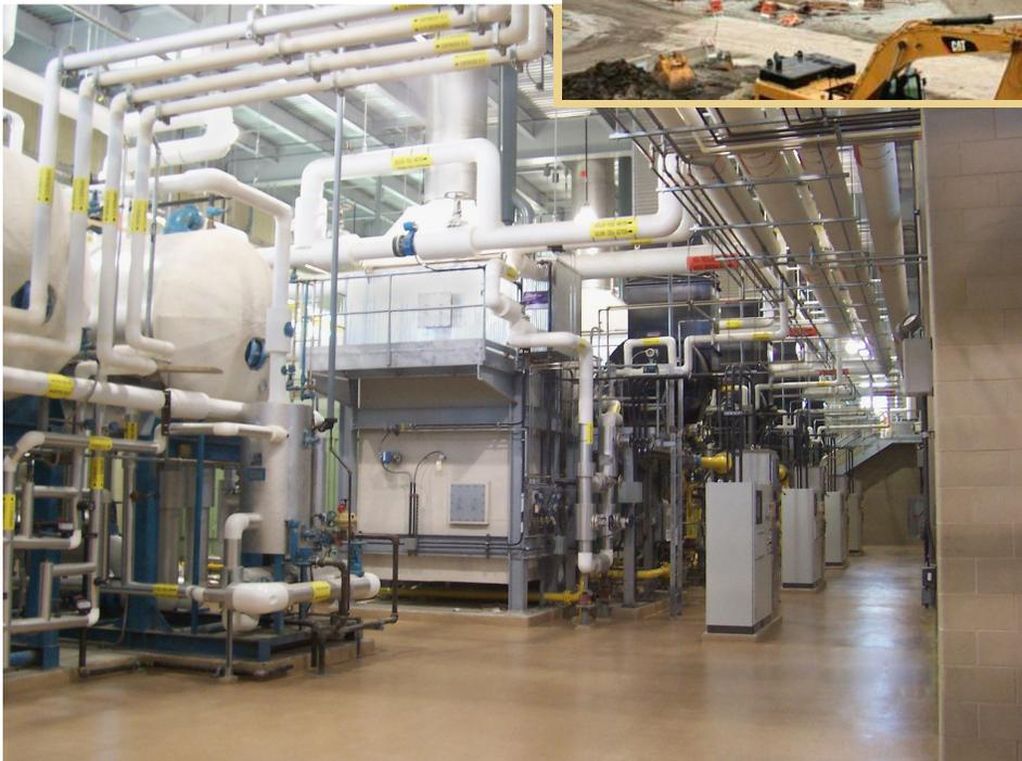
A new Central Boiler Facility has been constructed which will provide additional heating requirements with high efficiency boilers which will maximize digester gas usage.
