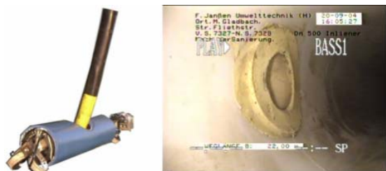
Figure C-27. Left: Packer. Right Renovated Lateral Connection (Originally a Protruding Lateral).
