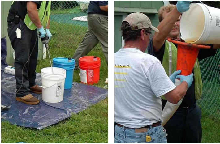
Figure A-36. Resin Mixing and Pouring into the Tube.
