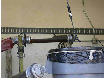
Figure A-27. Resin Cure. Left: Steam Hose Connected to the Bladder. Right: Steam Exiting at the Cleanout Near the House.
