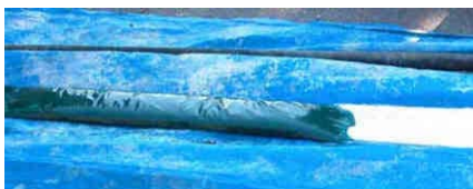
Figure A-52. Resin Progressing Through the Tube.
