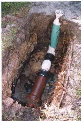
Figure A-80. Cleanout Installed in the Pit.
