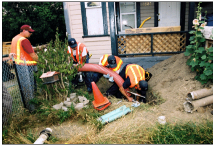
Figure A-7. The Crew Shooting the Liner into the Lateral.
