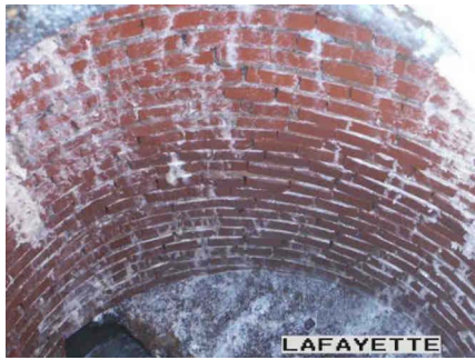
Figure A-101. Sealed Gaps on the Manhole Wall (Section #2).
