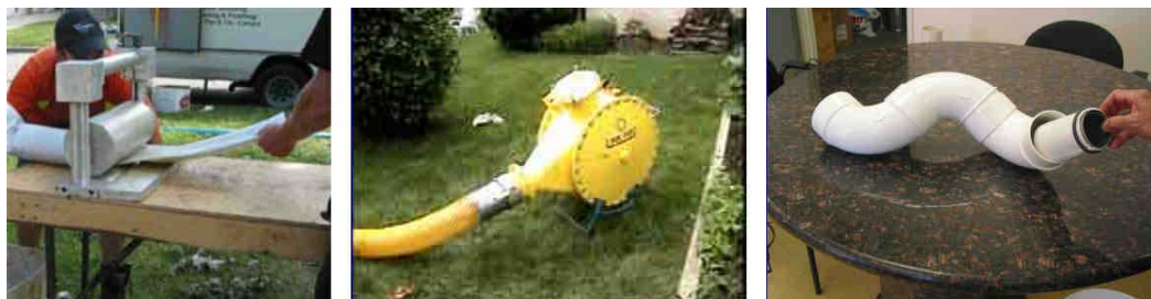
Figure C-1. Left: Roller System. Middle: Inversion Drum. Right: Drain Repair Sleeve in Elbows.
