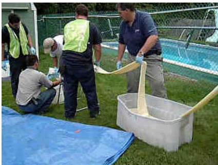
Figure A-39. Icing of the Liner to Prevent Premature Resin Curing.
