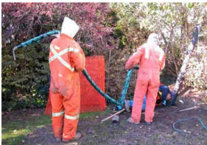
Figure A-56. Carrying the Liner/Bladder Assembly to the Excavation.
