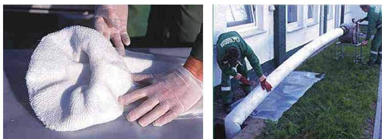
Figure C-5. InServ™. Left: Tube Material. Right: Insertion through a Small Pit.
