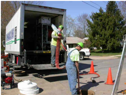
Figure A-25. Positioning of the Launcher. Left: Insertion through the Manhole. Right: Lateral CCTV Camera.
