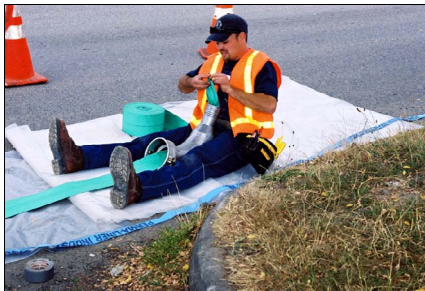
Figure A-8. Field Crew Member Preparing the Calibration Tube.
