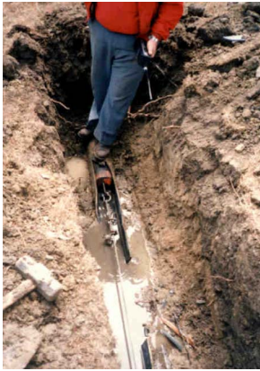
Figure A-130. Lateral Pulling Cable.
