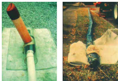
Figure C-13. Left: Loading of Inversion Device. Right: Inversion Device Ready for Installation.
