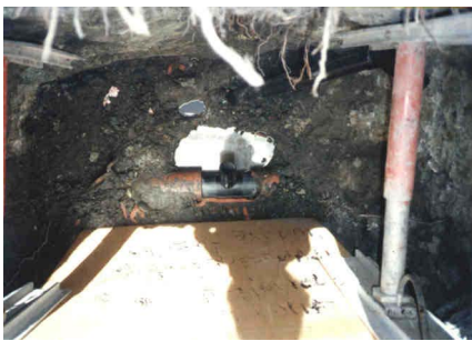
Figure A-131. Mainline Tee Ready for Lateral Connection—a View from Above.
