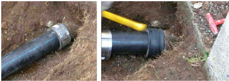
Figure A-76. Flexible Rubber Couplings with Stainless Steel Shear Bands.
