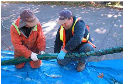
Figure A-55. Taping the Liner Tightly around the Bladder.
