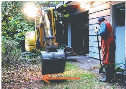
Figure A-47. Mark of Lateral Location Near the House.
