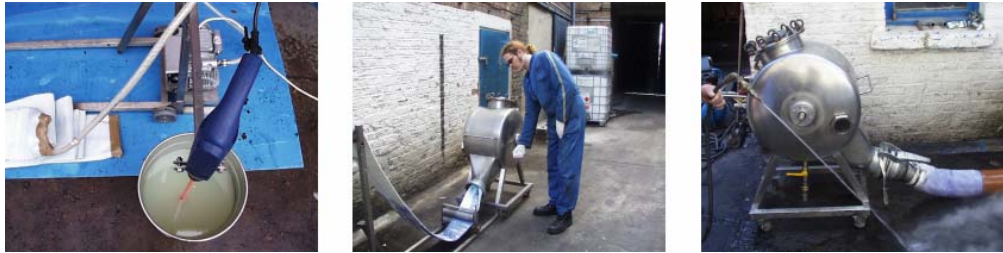
Figure C-2. Left: Vacuum Impregnation. Middle: Calibration Rollers. Right: Inversion Drum to Receive Warm Water.
