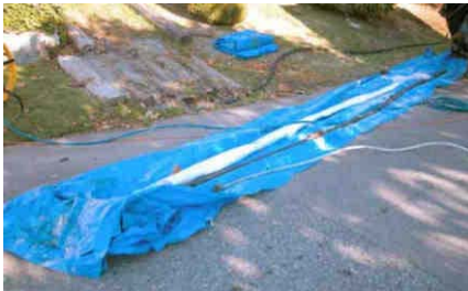
Figure A-50. Liner Tube Laid Out on the Ground.
