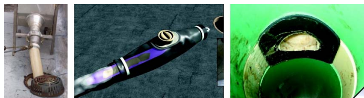
Figure C-14. Left: Inversion of MasterFlex through Cleanout. Middle: Insta T Inversion Device. Right: Insta T Installed.
