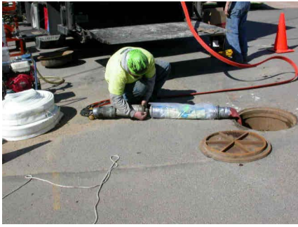
Figure A-24. Completing the Loading of the Launcher.
