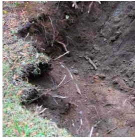
Figure A-66. Excavated Entry Pit.
