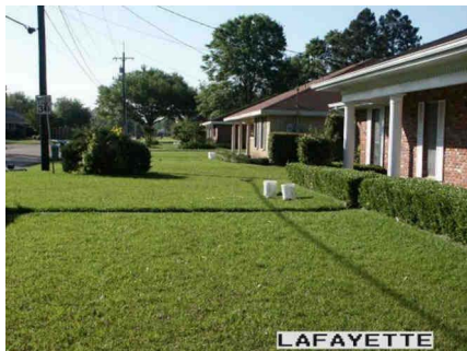
Figure A-94. Buckets Were Used for Adding the Water from a Nearby Hydrant Through the Cleanouts 47 .
