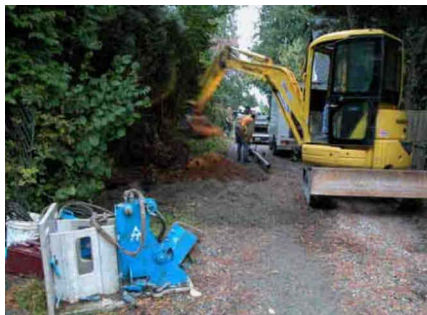
Figure A-67. Excavating of the Exit Pit at the Property Line.
