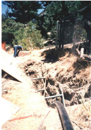
Figure A-128. One of the Additional Pits Excavated Along the Lateral.
