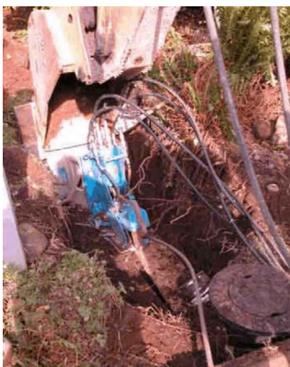
Figure A-74. Backhoe Assisting the Bursting in the Exit Pit.
