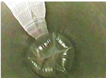
Figure A-26. Air Inversion of the Liner/Bladder Assembly the Lateral.
