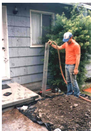
Figure A-125. Water Exfiltration Test Through Cleanout.
