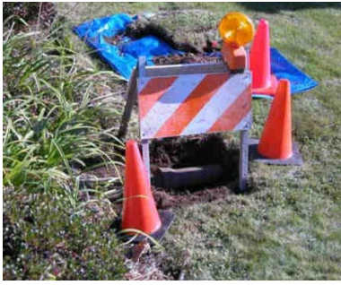
Figure A-49. Excavation Showing the Shallow Depth of Some Pipes.
