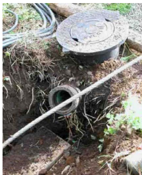
Figure A-68. Exposed Inspection Chamber.
