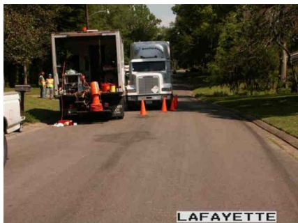
Figure A-92. Typical Site Setup Showing Tanker in the Background and Truck with Equipment in the Front.
