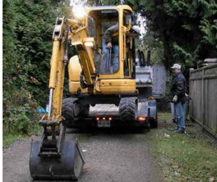
Figure A-62. Mini-hoe Trailed to the Site.
