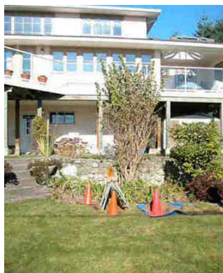
Figure A-48. Retaining Wall Near the Lateral Made Pipe Bursting Unsuitable.
