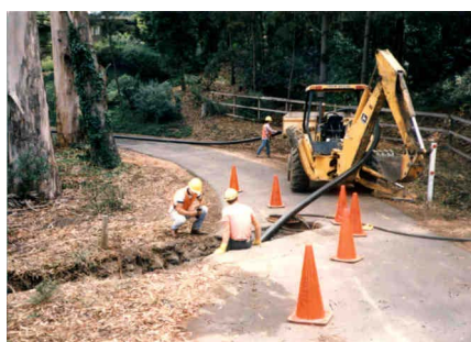
Figure A-126. Entry Pit at Lateral-to-Mainline Connection.
