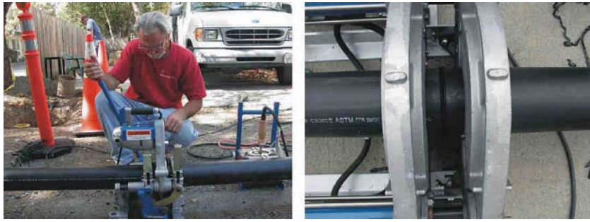
Figure 5-34. Pipe Fusing. Left: Cutting Pipe in the Jig. Right: Heated Pipe Ends Pressed Together (Tric Trenchless Inc).
