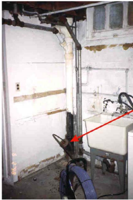
Figure 3-21. Lateral CCTV Inspection from a House Basement (City of Salem, OR).
