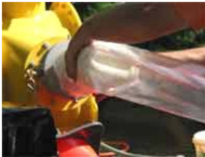
Figure 5-18. Inversion of Preliner (Link Pipe, Inc.).
