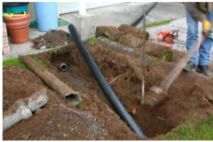
Figure A-75. Replacement Pipe Pulled in Place (Entry Pit Shown).
