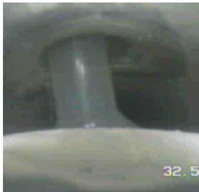
Figure A-45. Packer Deflation After Completed UV-light Resin Cure.
