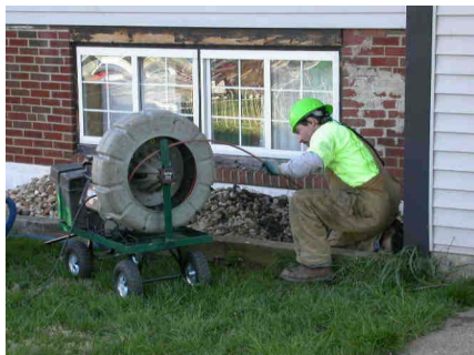
Figure A-20. Inserting the Lateral CCTV Camera into the Lateral.
