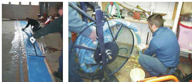
Figure C-3. Left: Liner Preparation. Right: Liner Insertion.
