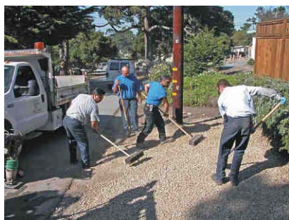
Figure 5-40. Surface Restoration (Tric Trenchless Inc).
