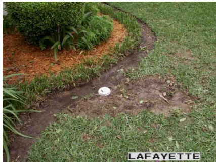
Figure A-91. Newly Installed Cleanout Close to the House.
