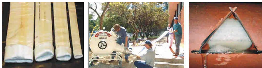
Figure C-8. Left: Liners 8" through 2". Middle: Preparation for Air Inversion. Right: Liner in Broken Pipe Sample.
