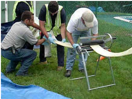
Figure A-38. Calibration Rollers for Even Wall Thickness of the Liner.
