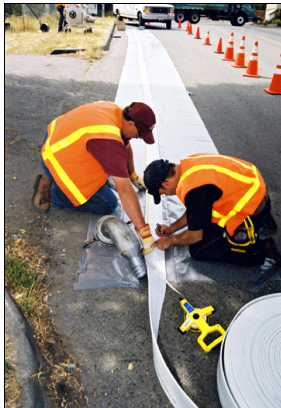
Figure A-4. Measuring the Length of Liner to Be Installed.
