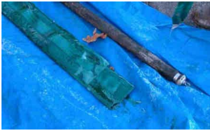
Figure A-54. The Bladder alongside the Prepared Liner.
