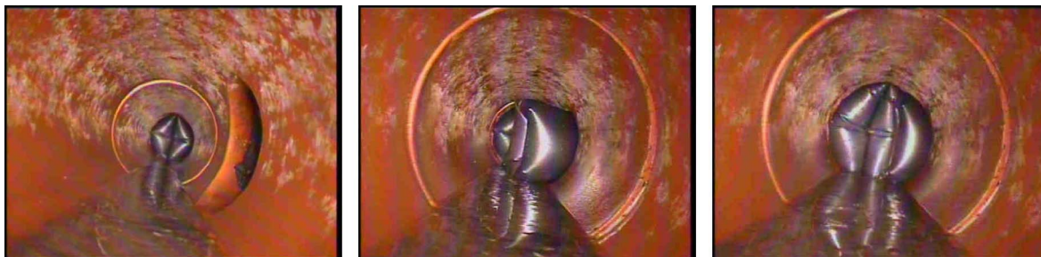
Figure A-113. Left: Lateral Bladder Retracted to Allow CCTV Camera to Pass. Middle: The Lateral Bladder Extended Again to Protrude as the Mainline Bladder was Approaching. Right: Mainline Bladder Inverting Past the Lateral Bladder.
