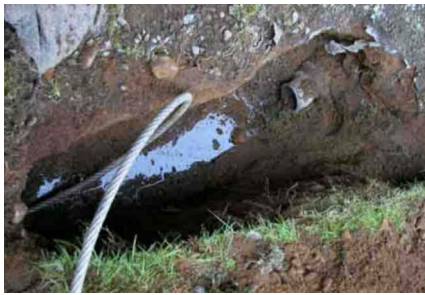
Figure A-73. Entry Pit Showing the Pulling Cable and Cut-off Section of the Lateral Near the House.
