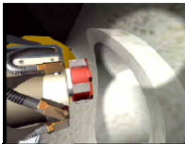
Figure C-28. Left: KA-TE Robots. Middle: Grinding Protruding Lateral. Right: Close-up of Grinding at Lateral Connection.
