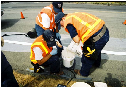
Figure A-3. Measuring the Pre-determined Amounts of Resins (Parts A and B). A Digital Scale Was Used for Accuracy.
