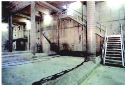
Figure 1-4. Peak Flow Storage Facility (Victoria, B.C., Canada).
