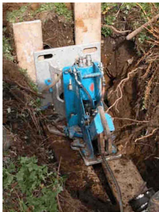
Figure A-70. Winch in the Exit Pit.
