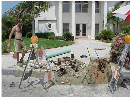
Figure A-84. Excavated Pit.
