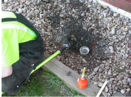
Figure A-19. Cleanout Ready for Pipe Cleaning.
