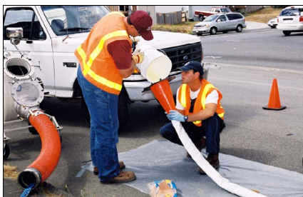
Figure A-5. Pouring the Pre-determined Amount of Resin into the Liner.
