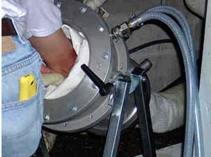
Figure A-40. Feeding the Liner into Inversion Gun.
