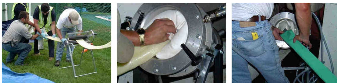
Figure C-7. MaxLiner. Left: Calibration Rollers. Middle: Liner Air Inversion with Liner Gun. Right: Bladder Inversion.
