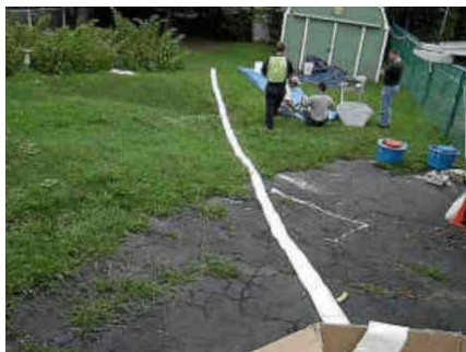
Figure A-35. Liner Tube Getting Ready for Wet Out.
