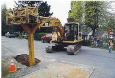
Figure C-17. Buno B-100 Pipe Bursting/Slip Lining Machine.
