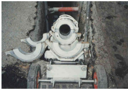
Figure A-127. Fuse Welding Machine.
