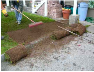
Figure A-60. Surface Restoration Underway.
