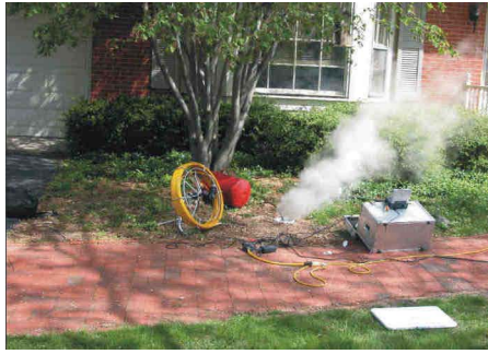
Figure A-27. Resin Cure. Left: Steam Hose Connected to the Bladder. Right: Steam Exiting at the Cleanout Near the House.
