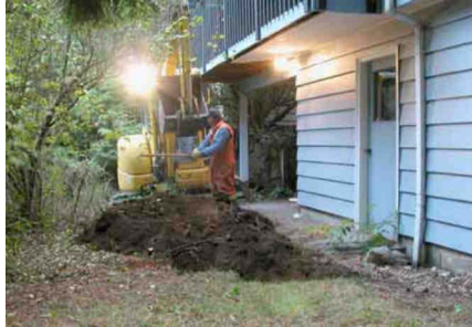
Figure A-65. Excavating of the Entry Pit Near the House.
