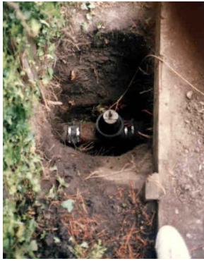
Figure A-132. Test Plug in the Lateral at the Property Line.
