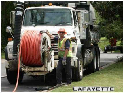
Figure A-93. Jetting Truck.
