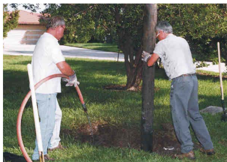
Figure 3-9. Hydro Excavating of a Cleanout Pit (City of Sarasota, FL).
