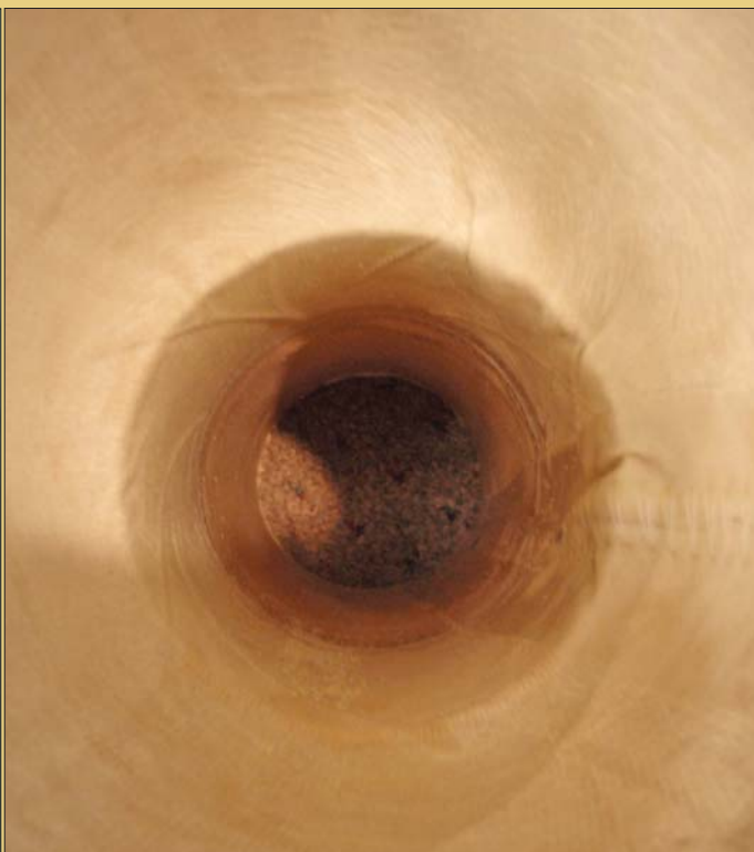
Cured-in-place (CIP) lateral lining is one of the most widely used lateral rehabilitation methods.
