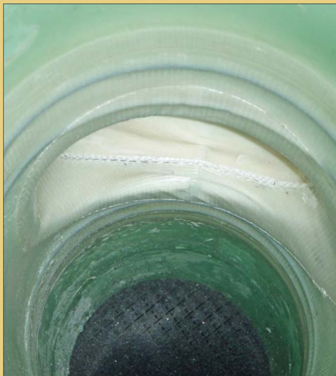
Cured-in-place (CIP) lateral lining is one of the most widely used lateral rehabilitation methods.
