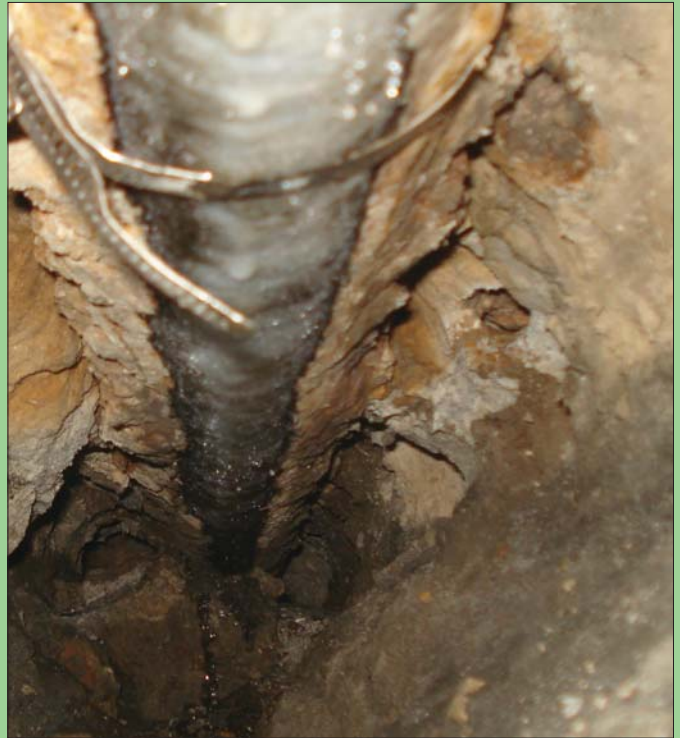
U.S. laterals are past their lifespan and trenchless professionals say they are a leading contributor to infiltration.
