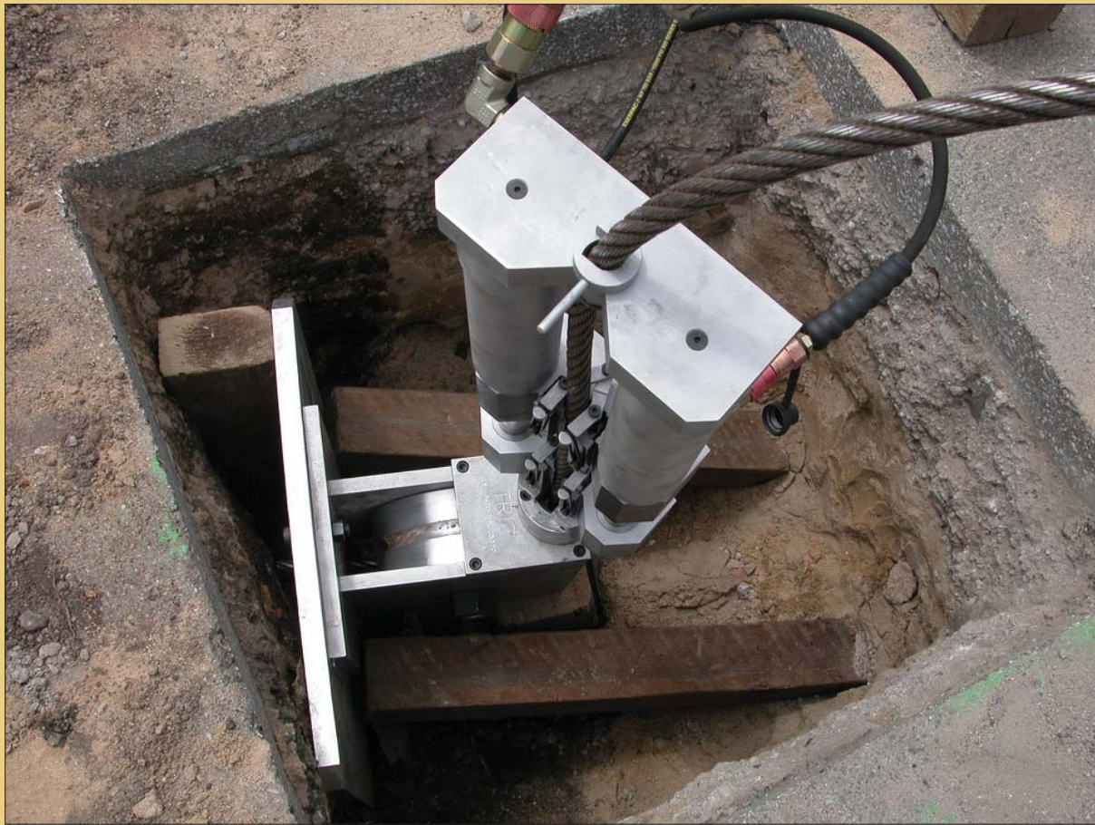
Lateral bursting is suitable for structurally damaged laterals on the verge of collapse.
