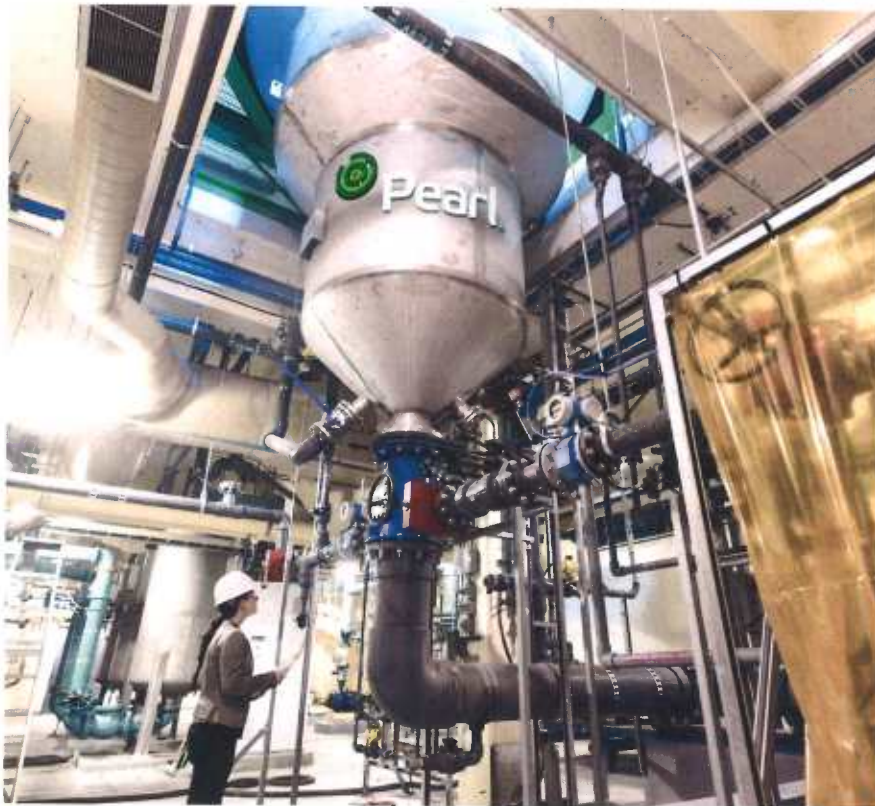
Figure 1: Photo of Ostaria nutrient recovery facility in Saskatoon Using Ostaria's Pearl 2000 system, Saskatoon's nutrient recovery facility has an annual production capacity of 730 metric tons of Crystal Green fertilizer, and the City receives revenue from the sale of the Root-Activated™ fertilizer.
