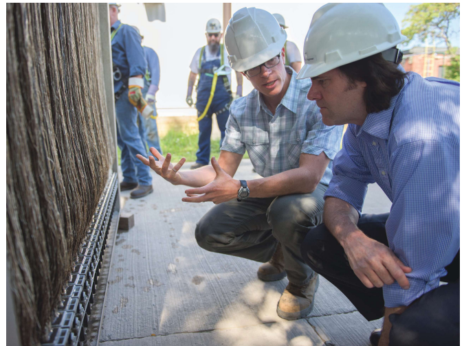
Careful consideration: MWRD is piloting GE's ZeeLung membrane-aerated biofilm reactor.
