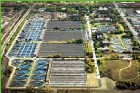
The Terrence J. O'Brien Water Reclamation Plant in north suburban Skokie treats much of the wastewater produced on the north side of Chicago and the city's near northern suburbs.
