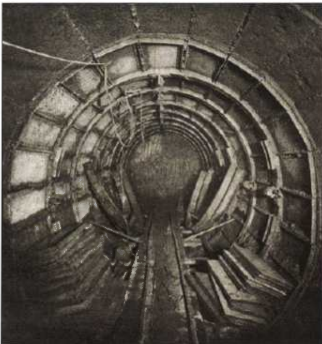
Figure 3. Cross-section of Blue Island Avenue Tunnel, during and after initial construction
