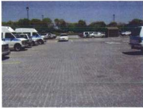
(c) Permeable Pavers
