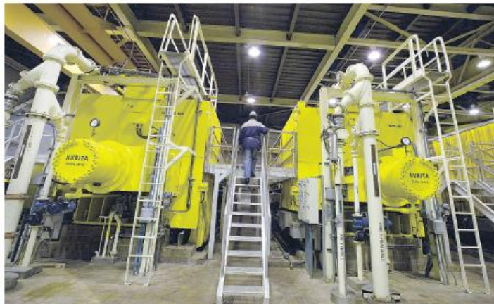
A city worker climbs onto the huge bank of racks that dry the sludge created as millions of litres of waste water are cleaned daily at the Montreal sewage treatment facility. ALLAN McINNIS/MONTREAL GAZETTE FILES
