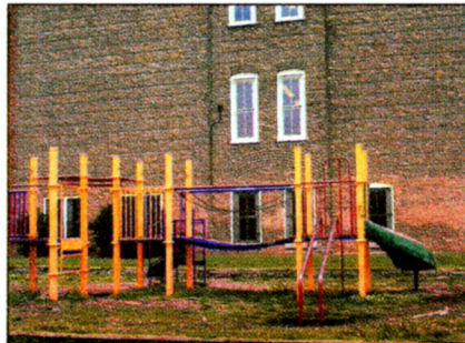
Old & dilapidated playground equipment is being replaced in a state-of-the-art exercise & recreation area at Leland School as part of an innovative campus redevelopment. (Photo by Brad)
