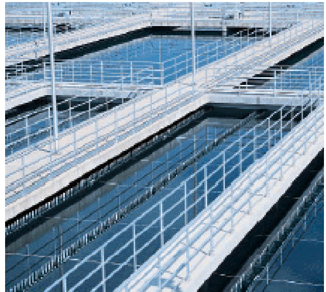
Chlorine Contact Tanks
