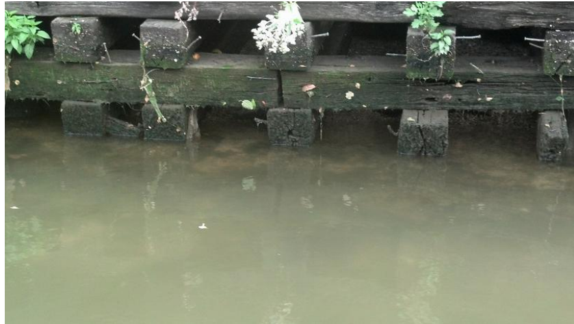
Railroad tie structure
