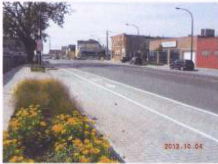
Planter Box Alongside Permeable Pavers in Bike and Parking Lane on Blue Island Ave.
