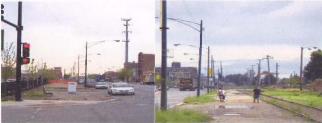
FIGURE 2: TWO STREET-LEVEL PHOTOGRAPHS SHOWING EXISTING CONDITIONS IN THE STUDY AREA ALONG CERMAK ROAD PRIOR TO THE START OF THE PROJECT
