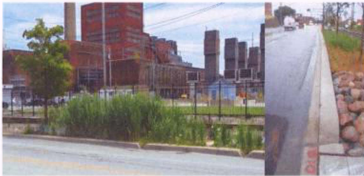
Bioswale on Cermak – Roadside view
