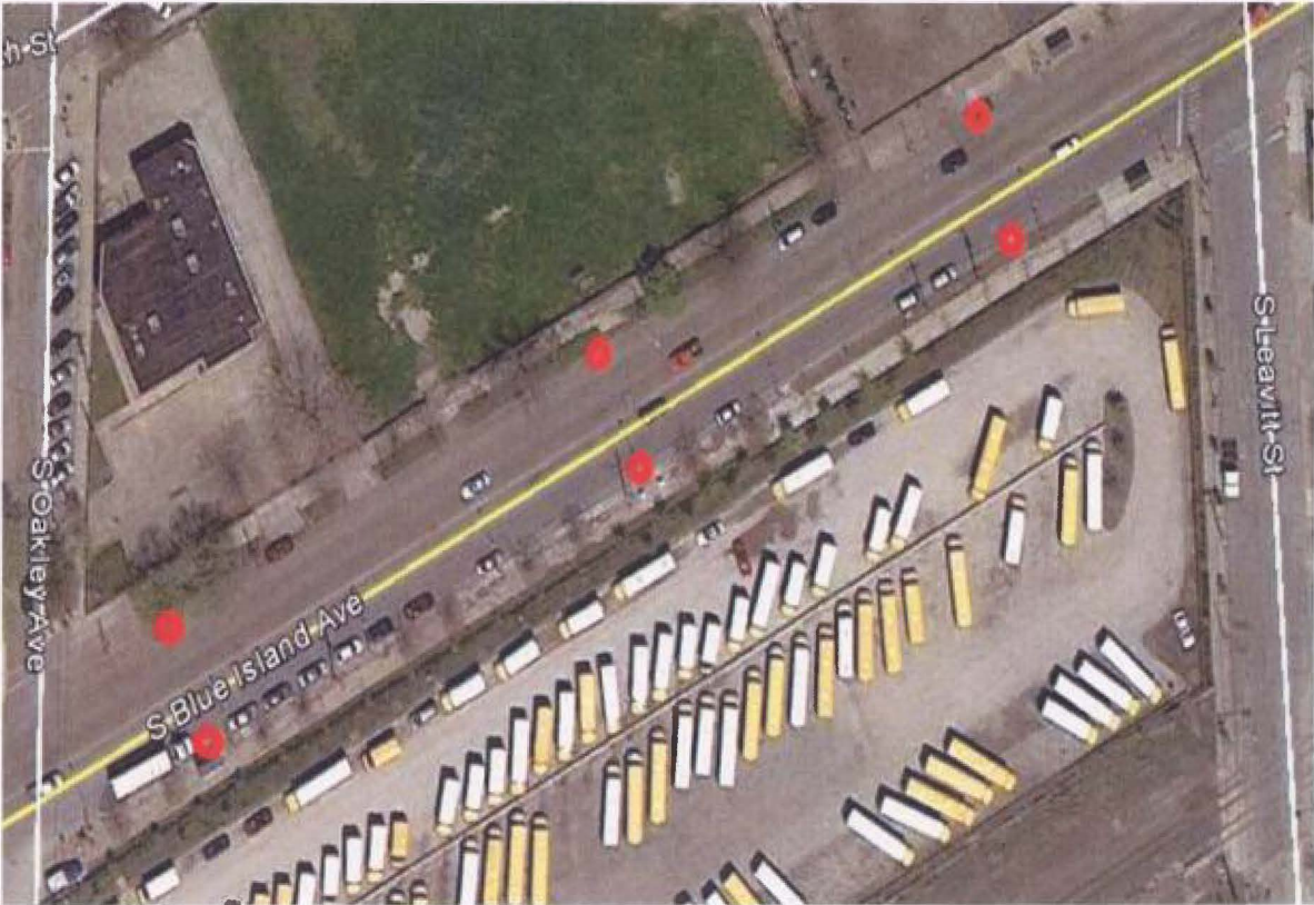
The Catch Basins
