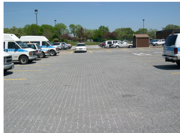
(c) Permeable Pavers
