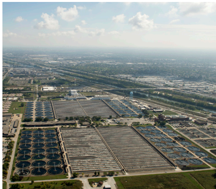
Stickney Water Reclamation Plant with the Chicago Sanitary and Ship Canal
