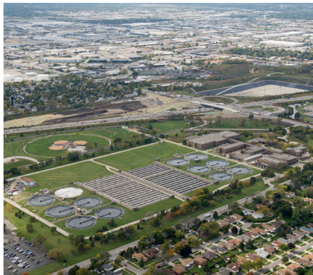
Kirie Water Reclamation Plant
