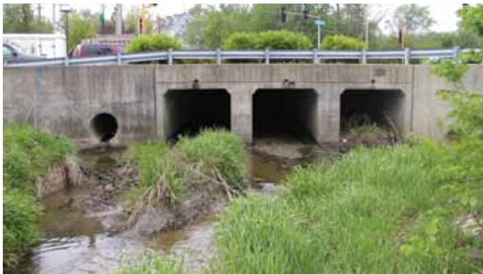
The culverts shown are located just upstream of the Margreth Riemer Reservoir in Palatine. Shown are before and after photographs of maintenance performed by the Palatine Park District. It is important that the debris be removed from waterways to allow for proper conveyance of the waterway and to prevent blockages which can result in flood damage upstream.
