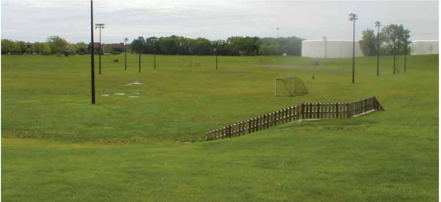
The Wilke Kirchoff Reservoir is located in Arlington Heights and provides 33 million gallons of stormwater storage. When not providing flood control benefits, this dual purpose facility can be utilized for recreational purposes.
