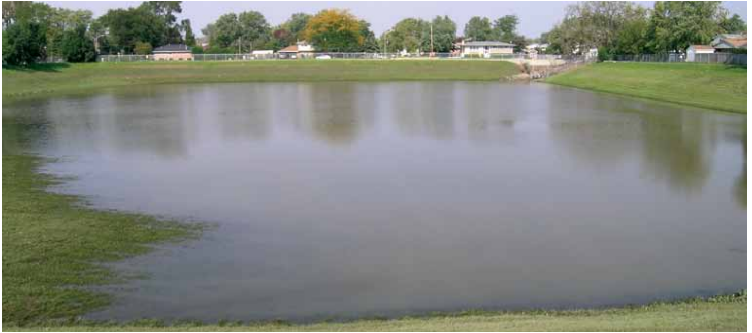
The Melvina Ditch Reservoir after a storm. The reservoir provides flood protection in the Cal-Sag watershed.
