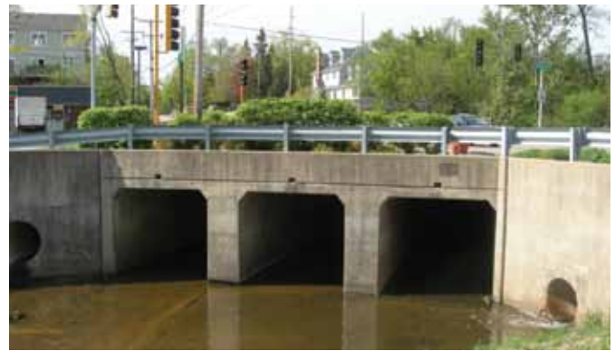
The culverts shown are located just upstream of the Margreth Riemer Reservoir in Palatine. Shown are before and after photographs of maintenance performed by the Palatine Park District. It is important that the debris be removed from waterways to allow for proper conveyance of the waterway and to prevent blockages which can result in flood damage upstream.
