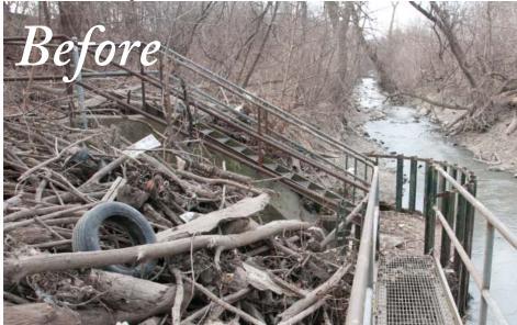
This photo was taken prior to the beginning of the project in January. During and after heavy storms, MWRD staff frequently cleared debris from the drainage structure in the foreground to allow for efficient drainage & flow away from the area.
