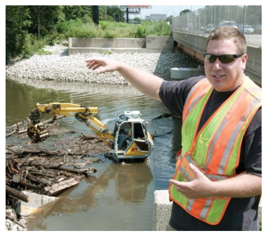
SSMP manager Brian Levy at a project site in Maywood discussing the methods employed by his crews to secure debris and remove it from a large waterway. Large debris is removed from the SSMP project site near the County Circuit Courthouse in Maywood (I-290 is seen in the background). This project required two days of work and the crew removed approximately 160 cubic yards of debris.
